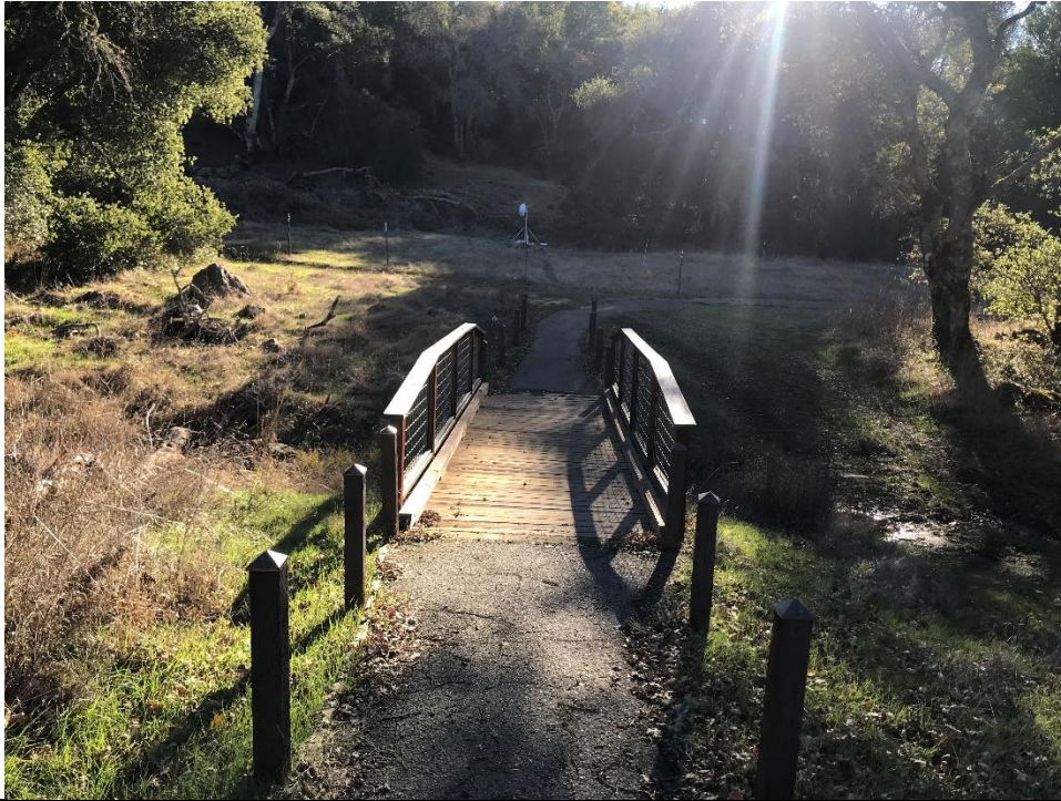
Photograph 1: View facing southeast of the seasonal drainage and pedestrian bridge near the center of the study area (December 29, 2020).
