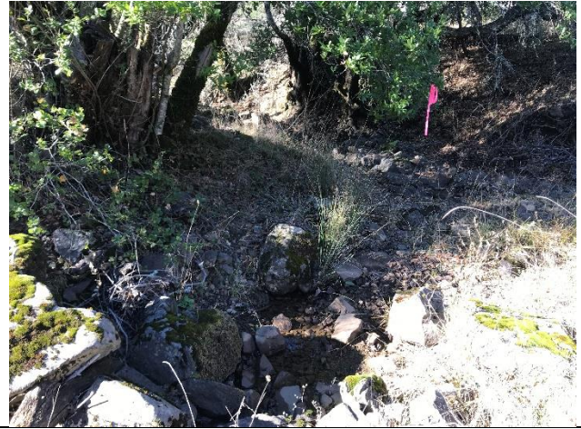
Photograph 5: View facing southwest of the seasonal drainage downstream of the pedestrian bridge (December 29, 2020).
